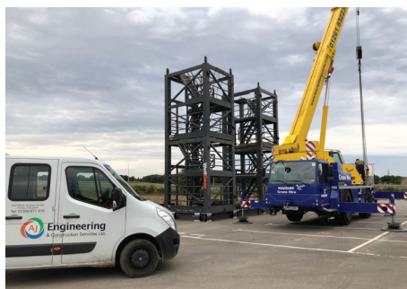
The frames partially completed
